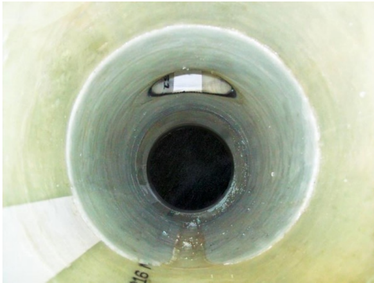
Completed lateral junction repair—LJR)
