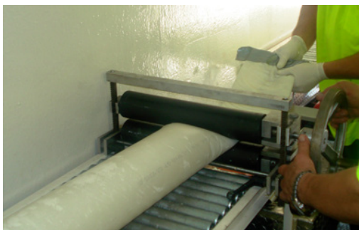
Liner impregnation onsite
